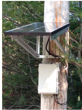
Fig. 3: Installation on a pole.
